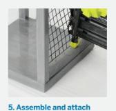
the hardware cloth panels. Using a staple gun, secure the top and bottom of the hardware cloth panels to the filler strips. Then nail the panels inside the lantern frame.
