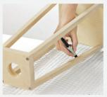
3. Size the hardware cloth. Use a permanent marker to trace the inside opening of the assembled frame onto the hardware cloth. Using wire cutters, cut three panels from the hardware cloth.
