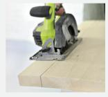
4. Prep the stretcher. Using a circular saw, rip 31/4 inches from the width of the  $2 \times 12$ stretcher board. Spread wood glue on each end.
