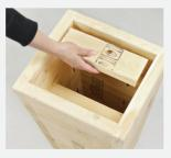
6. Create a pot ledge. To allow you to set a plastic nursery pot in the planter, mark its depth on the inside. Measure between the front and back walls at the mark; cut two scrap blocks to that length and bevel both ends. Wedge in the blocks, tapered side down.
