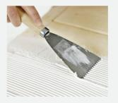
7. Skim-coat the walls. Apply flexible spackling to the exterior of the walls using a wide putty knife. Then pull a notched putty knife across the surface to create a ribbed texture, wiping the blade off after each pass and dipping it in water.
